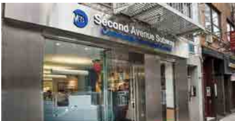
Figure 19 The Second Avenue Subway Community Information Center served as a community liaison office, educational center, and community meeting space during the construction of the subway line on the Upper East Side.
