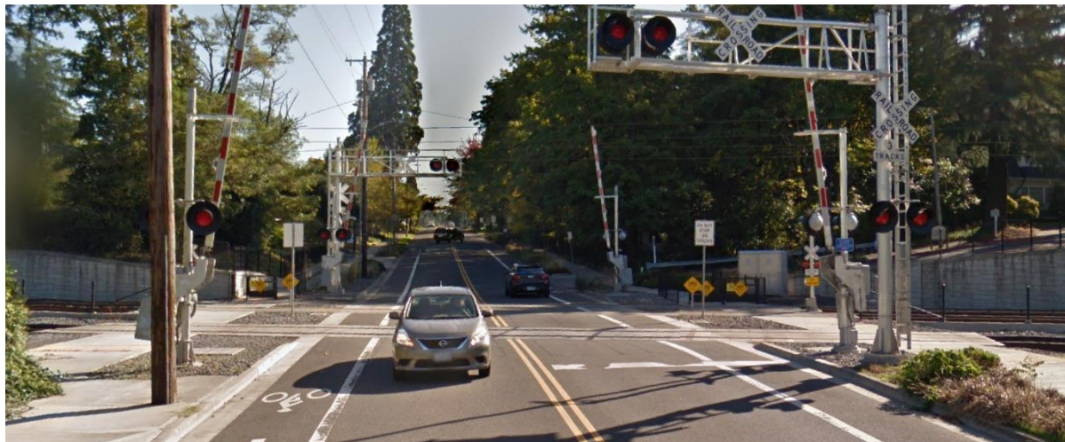
Figure 9: MAX at SE Harrison St. Grade crossing has quad gates, but no pedestrian control on near side (and only passive control, in the form of manually opened gates, on the far side). Speed limit for MAX is 30mph (Photo from Google Streetview).
